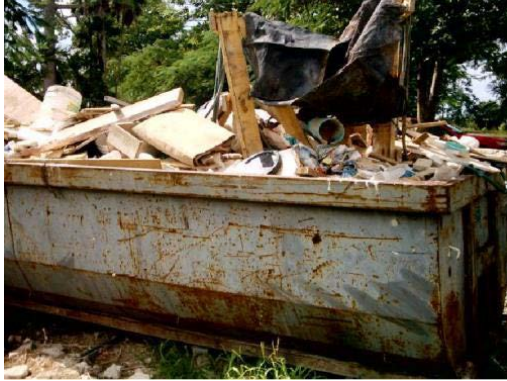
Unacceptable use of dumpster
